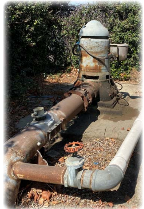
Metered Irrigation Well
